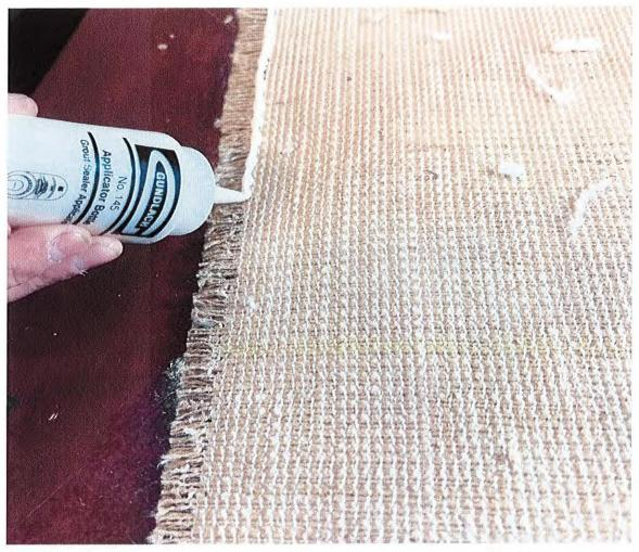
Run a bead of premium rubber-based latex on the backing, right on the edge of the chain stitch and exposed weft yarns.
