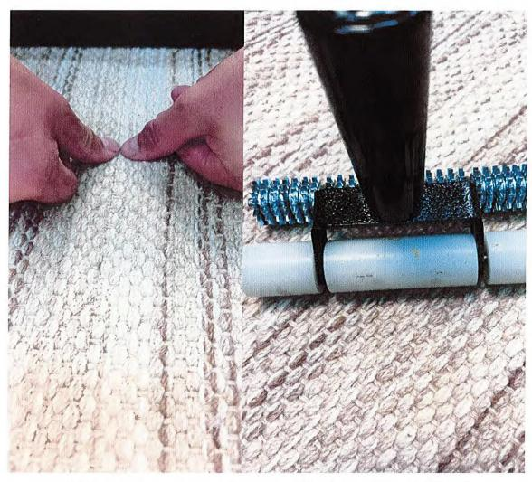
Always use a seam-roller and applied pressure to the edges of the seam tape to achieve maximum glue-transfer.
