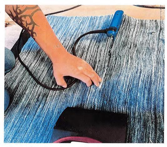
Use a premium low-melt seam tape with your iron set no higher than 2.5. Always use a seam roller and applied pressure for maximum glue transfer.
