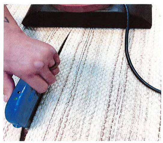
Using a premium low-melt seam tape and your iron set at no higher than 2.5, weld your two pieces together.
