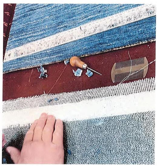
Fold the primary backing into the wet latex, applying pressure and smoothing it out.
