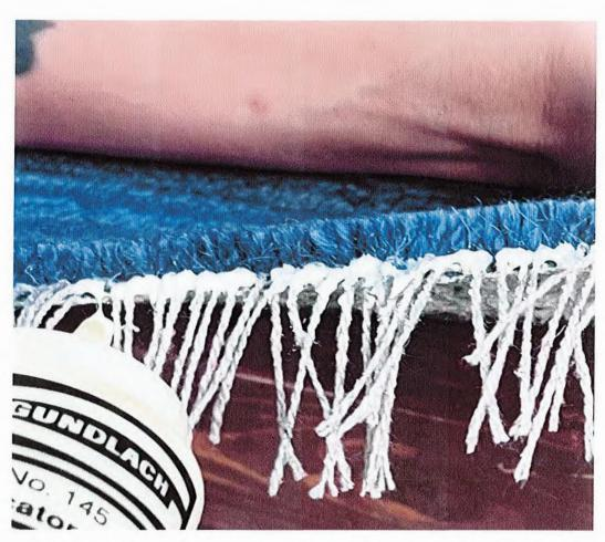
Apply a heavy bead of premium rubber-based latex on the seam edge, covering the chain stitch and folding the weft yarns down.
